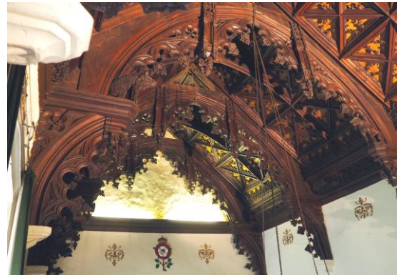
Part of the hammer beam roof of Weare Giffard Hall
